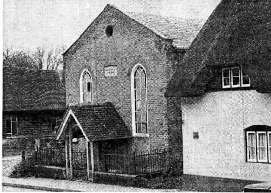
Wherwell's Wesleyan Chapel, due to be demolished to make way for a car park.
