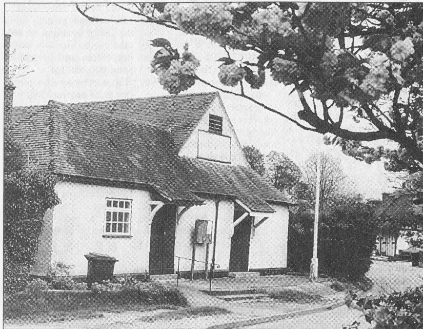
Staying put or coming down? Chilbolton Village Hall's future is in doubt J177/62/12
