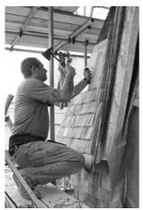
By the time you read this article the oak shingling on the spire should be finished, the renovated weathervane back in place and the dismantling of the upper scaffolding should have started. In addition the strengthening of the spire and bell frames will also have been completed. All in all very satisfactory progress, with the target date for completion of this first Phase still being around the end of October.
